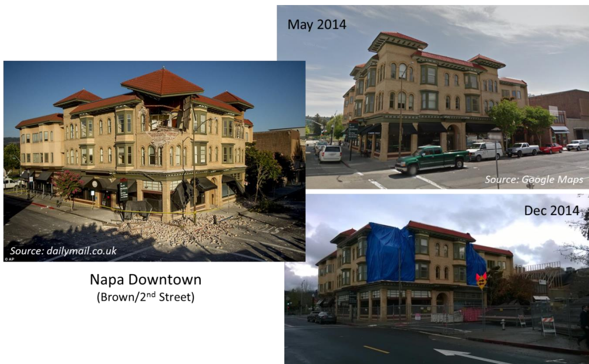
Figure 4: Damages to a masonry building in the historical Napa center (Brown St-2 nd St)
