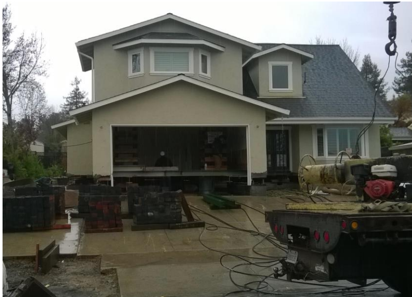
Figure 22 : Work in progress on a residence foundation affected by faulting, located on the primary fault trace A (close to NAPA30 waypoint, White Cliff Circle). The house has been uplifted for the repairing. Surface slip was measured to be around 10-15 cm.
