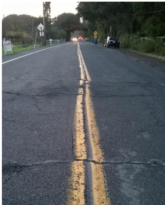
Figure 12: Right-lateral displacement (28 cm) of the Las Amigas road, on the southern section of the 'A' strand, cumulates on several parallel segments (NAPA18). At this place, afterslip is high (more than 90% of the net slip). Picture december 2014.
