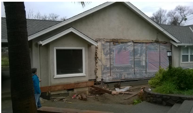
Figure 23 : Work in progress on a residence foundation affected by faulting, located on the secondary (distributed) fault trace C (close to NAPA2 waypoint). The wall has been destroyed by workers after the earthquake. A 5-6 cm Surface slip was measured on the close road pavement just after the earthquake.
