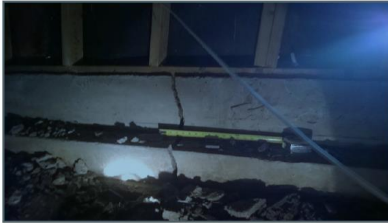
Figure 21 : Example of a strip footing foundation displaced by faulting (picture from Bray et al., 2014)
