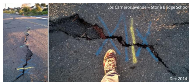
Figure 19: Field evidences of afterslip along the main trace. Top: Leaning Oak (NAPA29), northern section of main segment (left picture from UC Davis); Middle: Highway 12 (picture from Bray et al., 2014, GEER report), southern section of the main segment (NAPA23); bottom: Los Carneros avenue, southernmost part of this segment (NAPA19); blue and yellow lines were drawn on the fault rupture in the first hours after the mainshock and their later offset illustrates the postseismic slip (afterslip).
