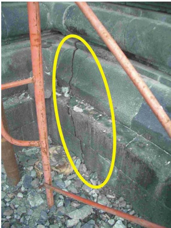
Fig. 6: Brahma temple: a NW-SE left-lateral fault cross-cutting the temple diagonally. A reinforced concrete wall surrounds the level below this floor. There was 4 mm left-lateral displacement.
